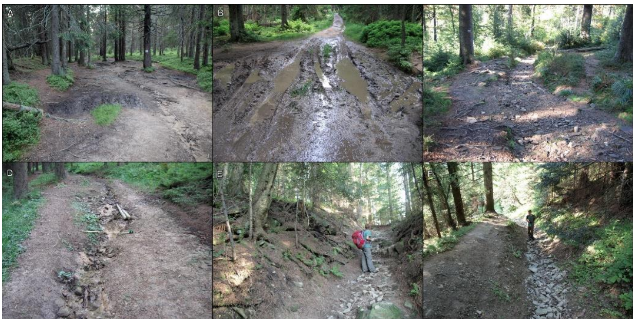
Fig. 1. Examples of trail impacts: (A) deposition of material due to improper trail drainage; (B) muddy section and water puddle; (C) exposed roots and rocks on the too-narrow section of the trail, forcing visitors to trample trail sides; (D) erosional rill along the trail tread; (E) deep erosional gully reaching bedrock; (F) erosional gully with exposed rocks: Due to uncomfortable walking condition, visitors created an informal path next to the designated trail.
